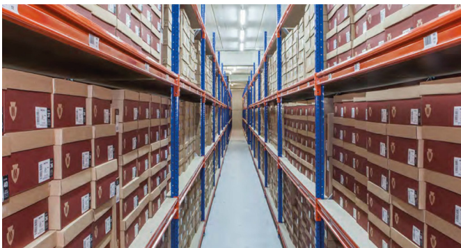
TUFF Longspan Shelving Units Client Installation
